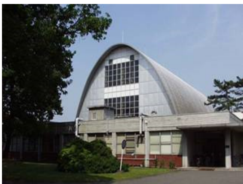
Gamma-ray irradiation facility building
