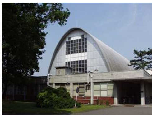
Gamma-ray irradiation facility building
