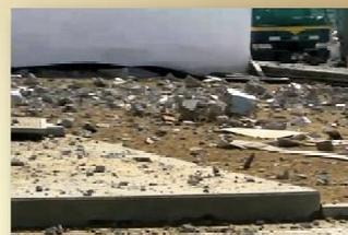
Concrete debris scattered with hydrogen explosion were the dominant gamma source for external exposure.
