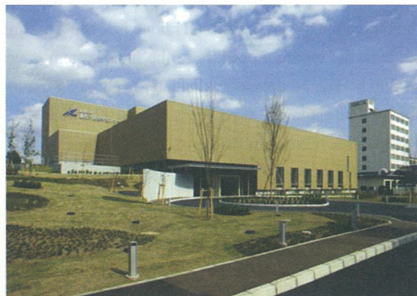
Fig. 2. Outside view of the facility
