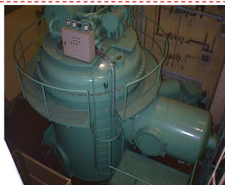
Electron accelerator (0.5~2.0 MeV, 0.1~30 mA)
